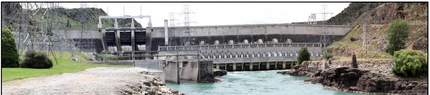
Figure 1 Contact Energy's Roxburgh Power Station, Roxburgh, New Zealand.
