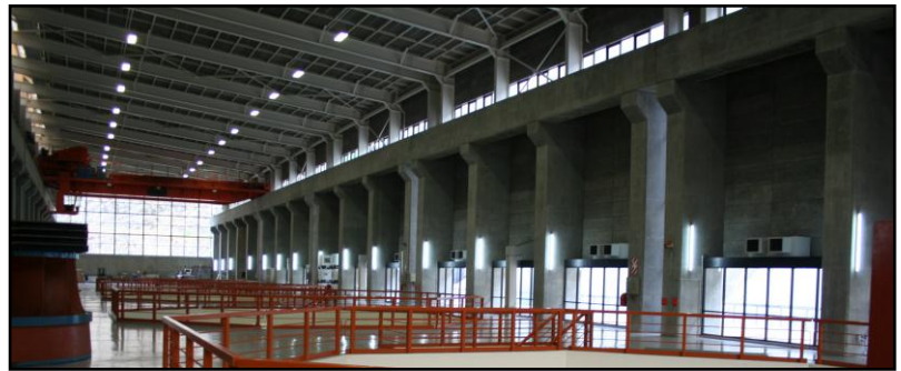
Figure 2 The Machine Floor at Clyde Power Station
