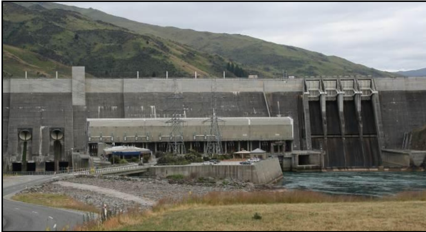
Figure 3 Contact Energy’s Clyde Power Station, Clyde, NZ.
